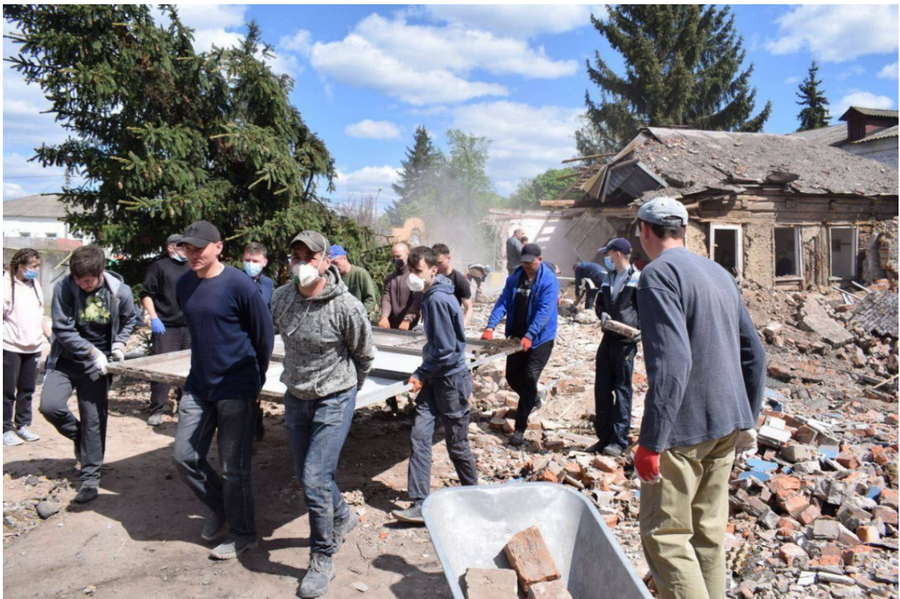
Photo by Dobrobat organization (volunteer construction battalion)
