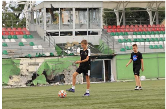
Kharkiv region: destruction of the Karazin University Stadium and training complex (Unifecht) Photo: Vlad Sakovych/HOWA
